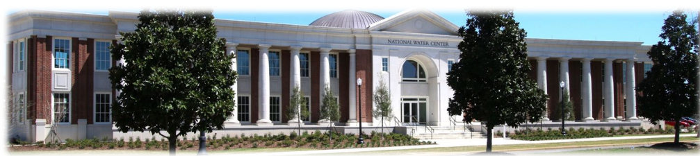
National Water Center - Tuscaloosa, AL
